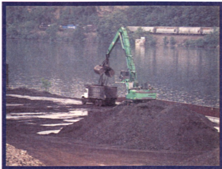
The SENNEBOGEN 870 M loads a truck with coal from the barge it is unloading at Lindy Paving's Neville Island Terminal dock. The 870 M can unload three barges in approximately 7 1/2 hours per day.
